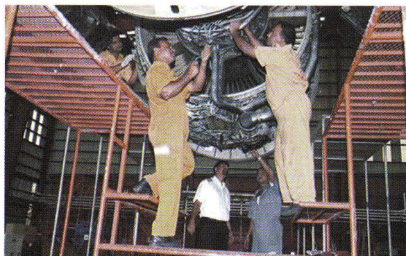
SL Engineering carries out first 4C5Y check on Airbus A340 in record time
